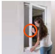
5. Press the sash completely into the upper corner of the frame and continue to hold the sash lifter in a vertical position.
