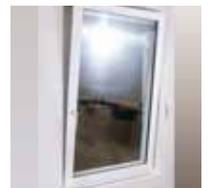
2. Do not force the window shut. The sash or fitting could be damaged. Leave the window tilted and turn the handle 90° in the direction of rotation.
