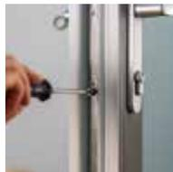
2. Then insert the key into the profile cylinder and turn the key 15°–20°. The cylinder can now be gently pulled out.
