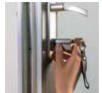
3. Insert the new cylinder. For this purpose, the cylinder must move smoothly and be seated in the fitting with as little tension as possible. If you have a security level 2 cylinder, make sure that the parts of the profile cylinder are on the intended side (outside or inside). The outside is marked.
